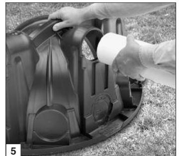
Insert inlet pipe.
