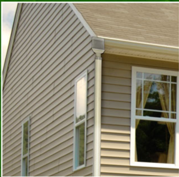
Debris strainer located at water source
